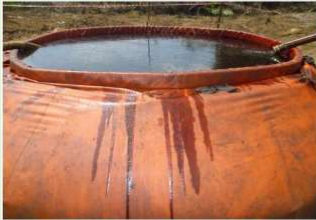
Mechanical Transfer/recovery of crude oil into fast tanks
