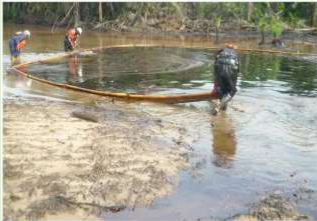
Containment of spilled crude for recovery at 20" Otumara-Escravos Trunkline spill site in Ugboegungun
