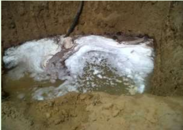
Application of OSE II in excavated pit
