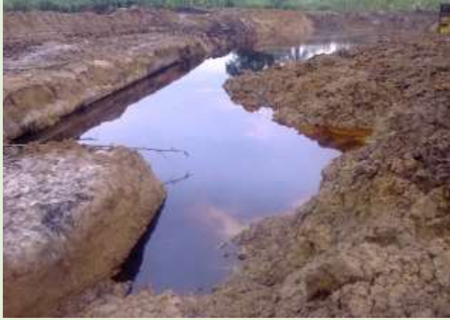
Excavated Ground Water trench with Free Phase crude before recovery and application of OSE II
