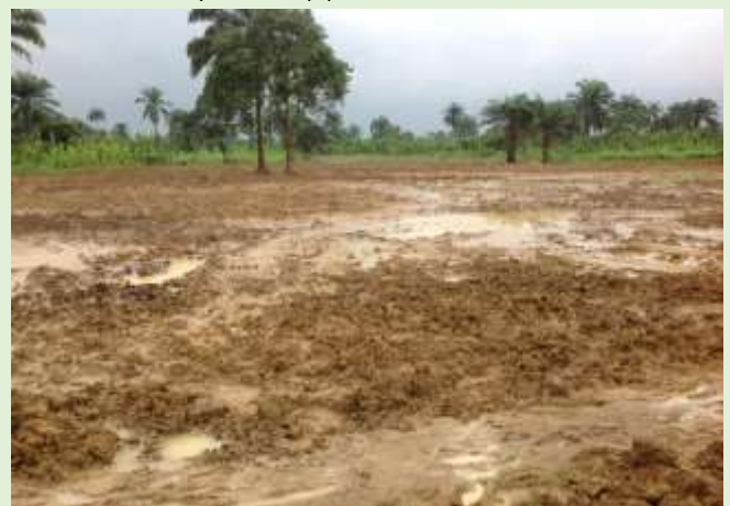
Overview of site after groundwater treatment with OSEII and backfilling of excavated pits
