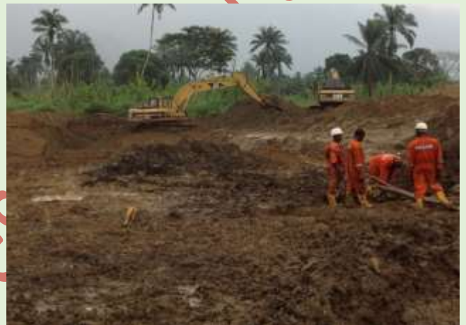
Mechanical Excavation of impacted area
