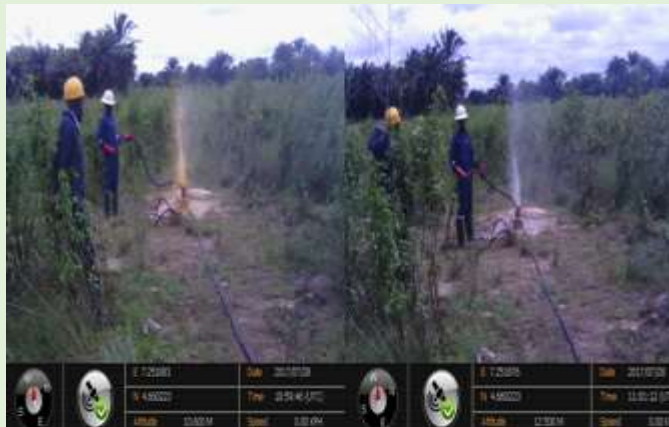
Flushing of Boreholes using Air compressor
