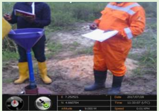
Conducting Falling Head test on site
