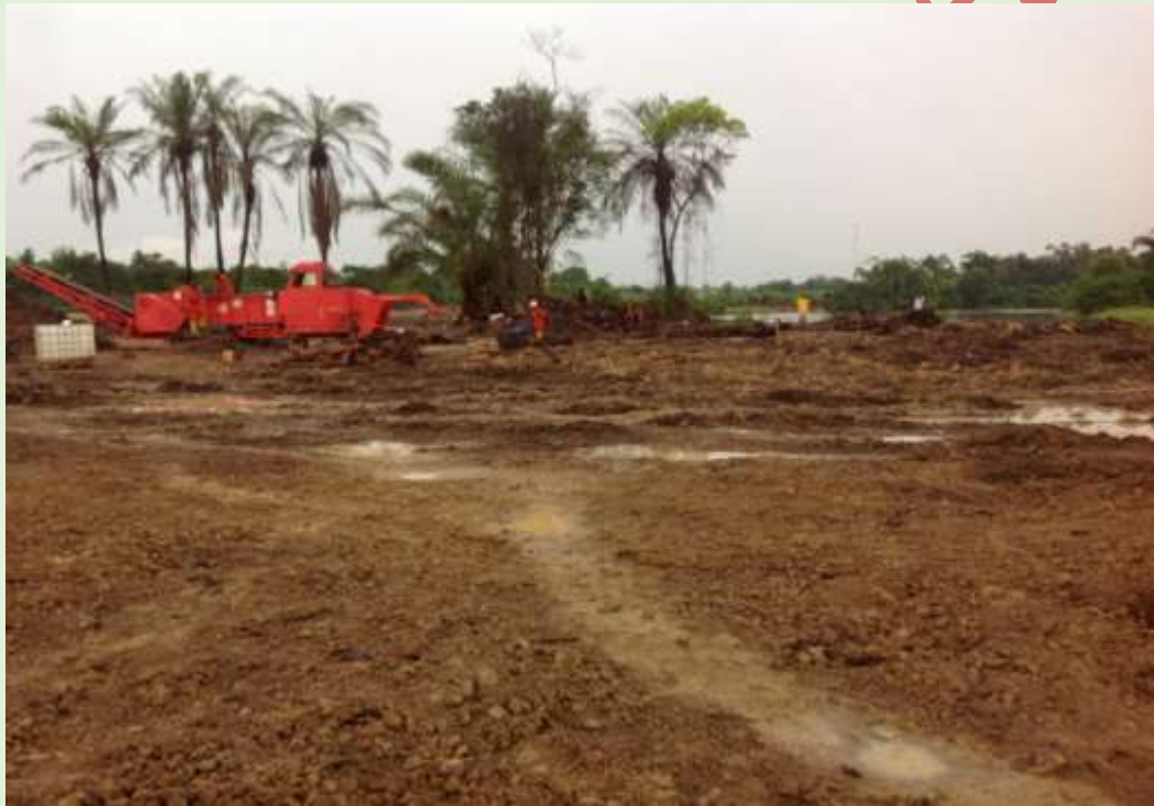
Overview of site after remediation and waste management
