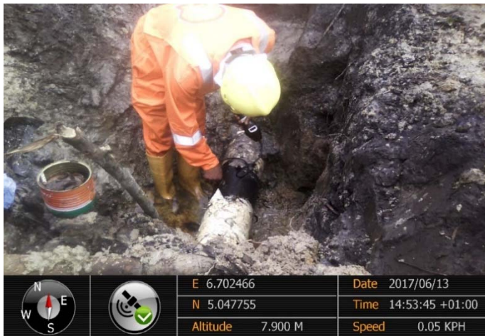
FIG 1: spill point showing bubbling crude oil.
