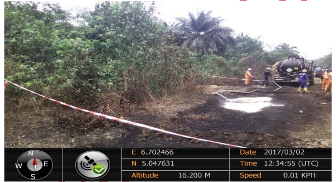
FIG 2: recovery of crude oil using vacuum truck.
