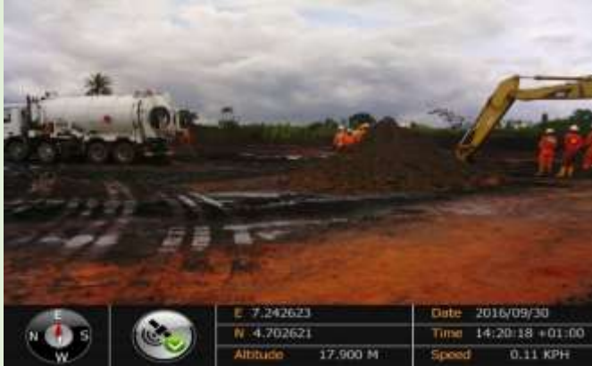
Fig 5: control release into vacuum truck
