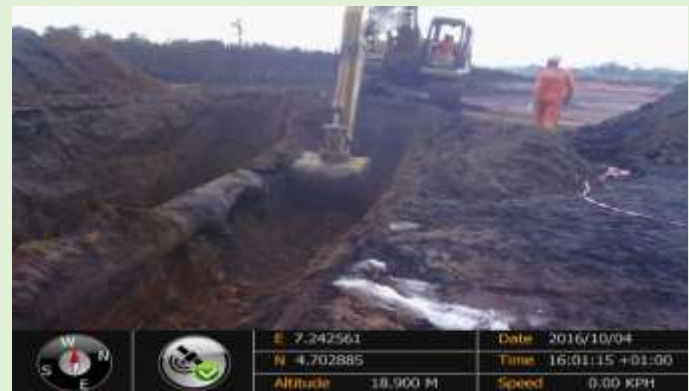
fig 4: excavating the spill point
