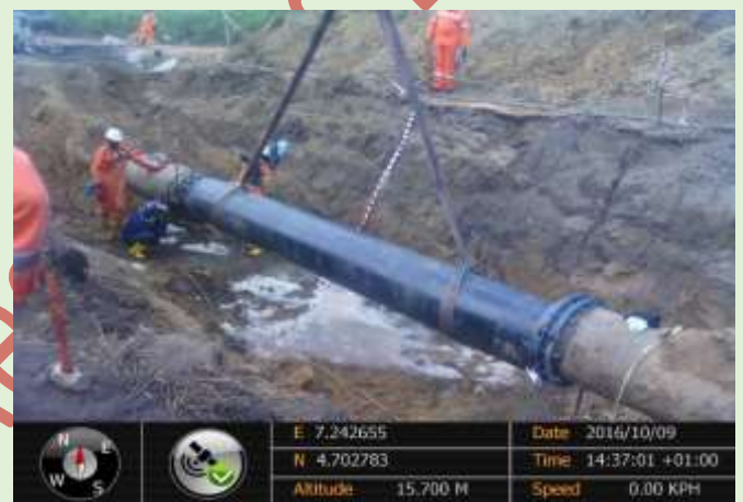
fig 8: sectional replacement ongoing
