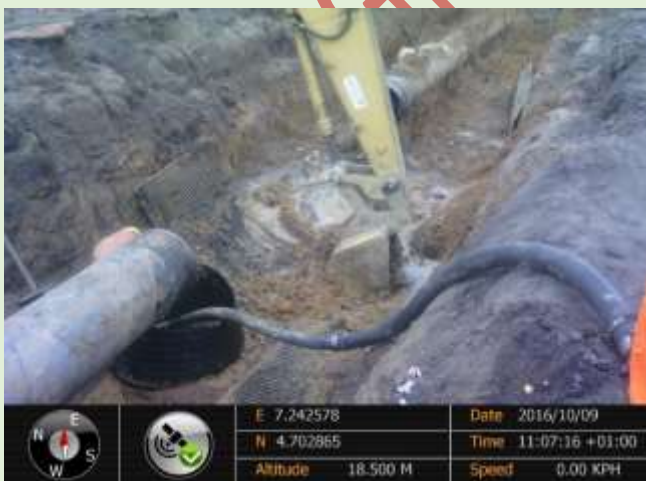
Fig 9: recovery from the source pipe
