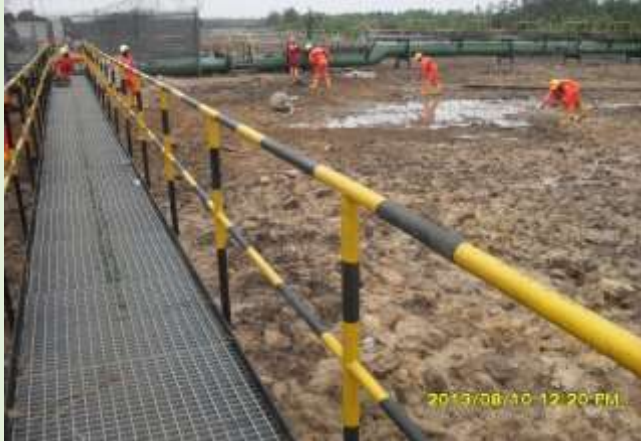
Homogenization of filled soil
