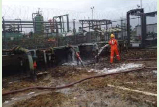
Flushing in progress
