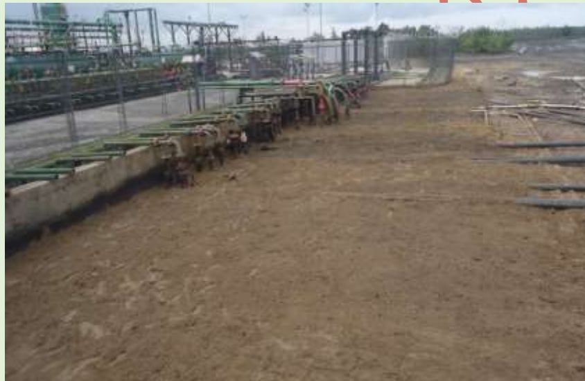
Overview of site after clean-up and remediation activities
