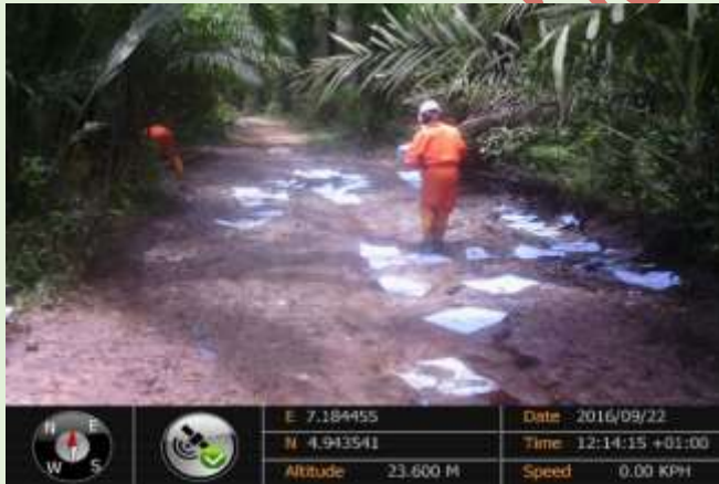
Fig 3: Mopping of Residual oil deft point.
