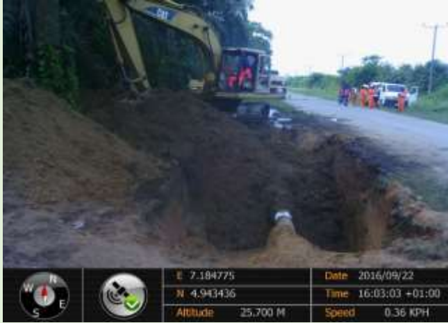
Fig 5. Back filling of excavated spill point
