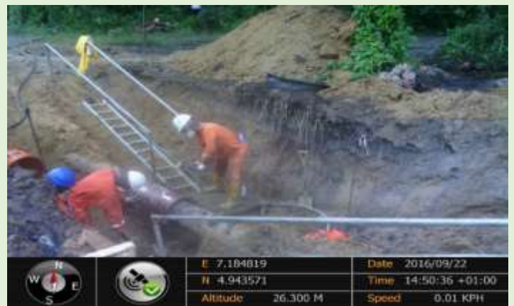
Fig 4: Repairs Ongoing on the deft point
