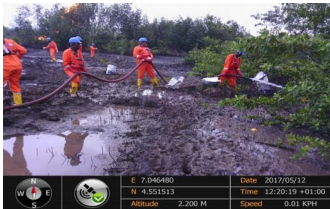
Plate 4: flushing of trap crude oil process
