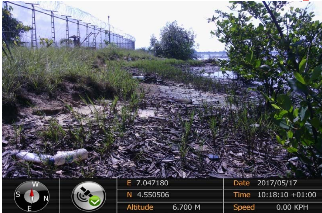
PLATE 1: INITIAL SITE PIC BEFORE WORK
