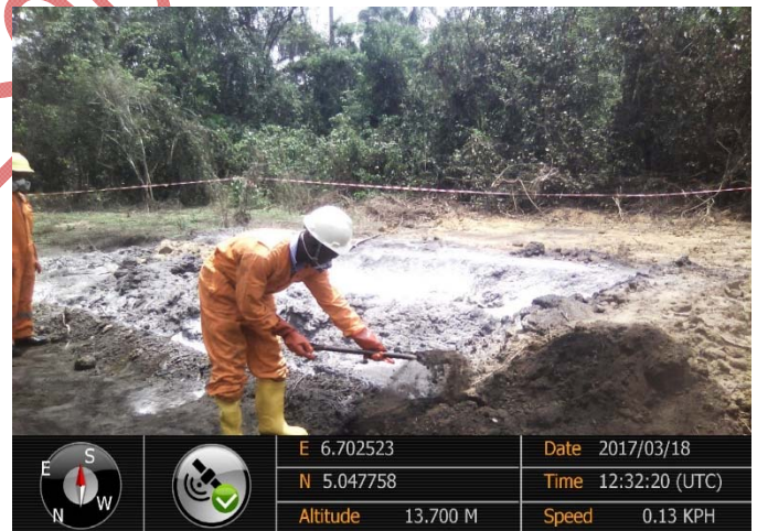
FIG 1: spill point showing bubbling crude oil. FIG 2: recovery of crude oil using vacuum truck.
