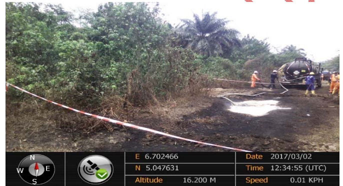
FIG 1: spill point showing bubbling crude oil. FIG 2: recovery of crude oil using vacuum truck.
