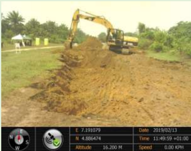
Plate 5: Mechanical tilling of delineated area
