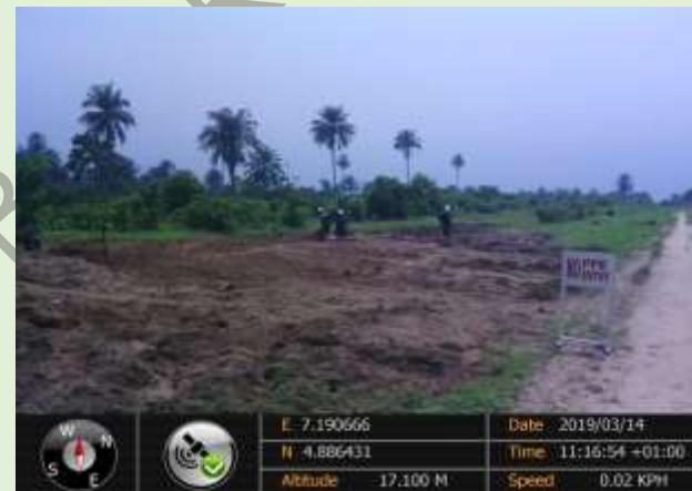
Plate 8: Back filling of excavated area
