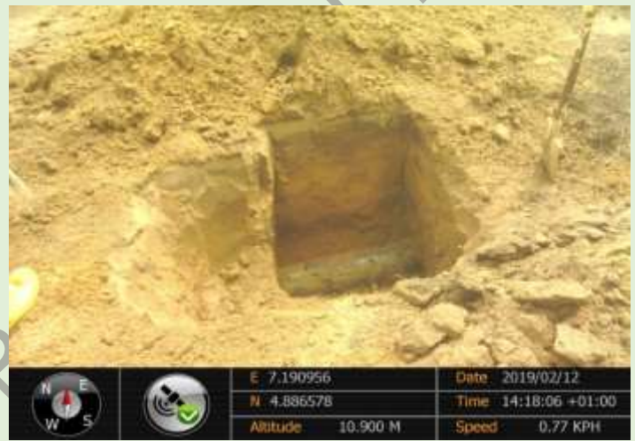
Plate 2: Probing for the pipeline
