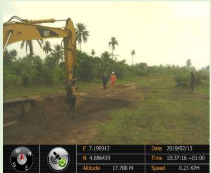
Plate 4: Mechanical excavation of the hot spot
